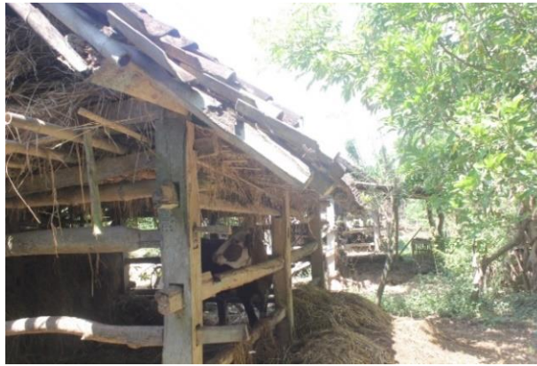
Figure 3. Constructing the Worms Cage
